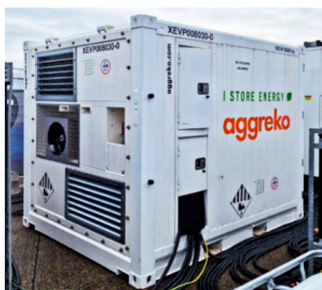
FIGURE 14: Example of a battery bank used to charge electric vehicles in Berlin. The battery bank charges slowly from the grid, but discharges quickly into the vehicles.
